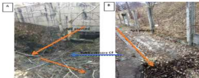
Fig. 3. Drainage channel A: in the right side of the ramp (drain pipe and chimney) and B: in the left side of the ramp, after undercrossing CF (chimney and collector ditch)
